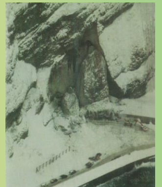
Collapse of Toyohama Tunnel
