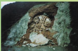
Tunnel Boring Machine
